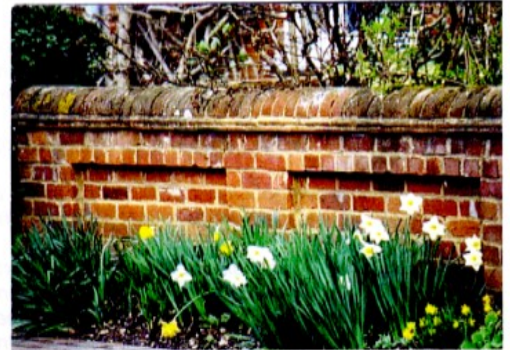
GOOD EXAMPLE OF A MODERN BRICK WALL USING TRADITIONAL MATERIALS AND DESIGN DETAILS
