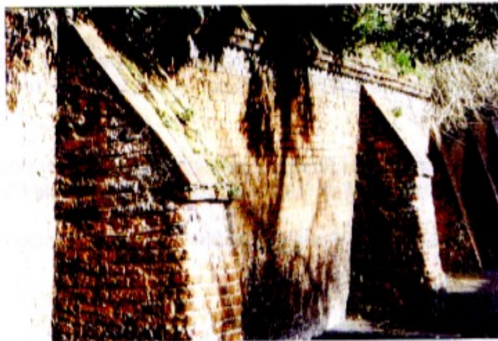
BUTTRESSES AND STRING-TOOTH BRICK COURSES CREATING STRONG VISUAL INTEREST IN A BOUNDARY WALL
