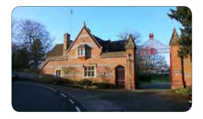
window. Toothed brick course at top of wall under shaped coping bricks. Square fluted multiple shaft central chimney. Stone copings on gable ends with stone finials. C20 extension to left.
